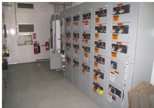
Siemens MARQ 21 Dual Breaker Feeder
